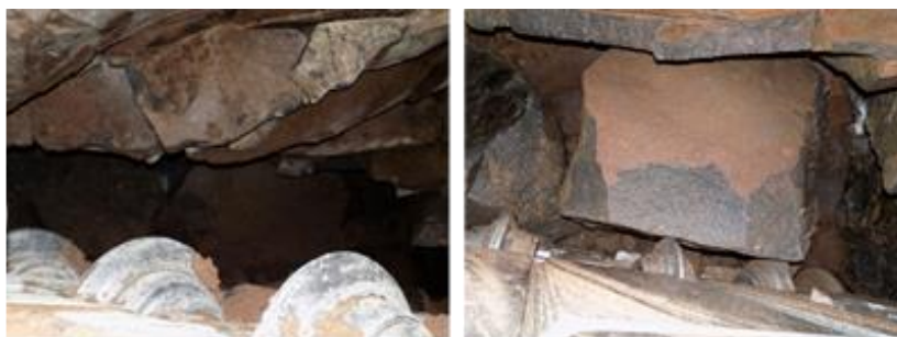
Figure 8. Block formation at the tunnel face.
