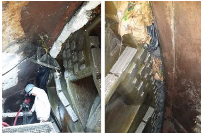
Figure 18. Intervention after stop of water inflow.
