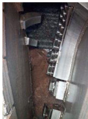
Figure 7. Mixed face conditions.
