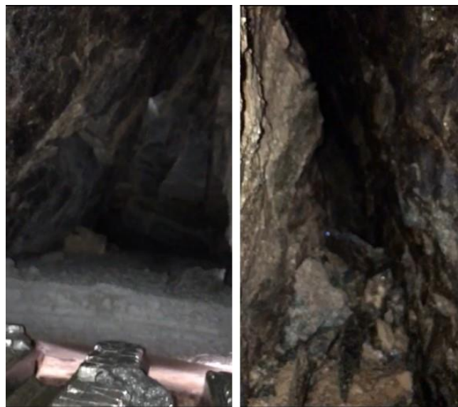
Figure 11. Encountered discontinuity in the rock mass (Left: view against drive direction above the shield; Right: view in drive direction at the face).
